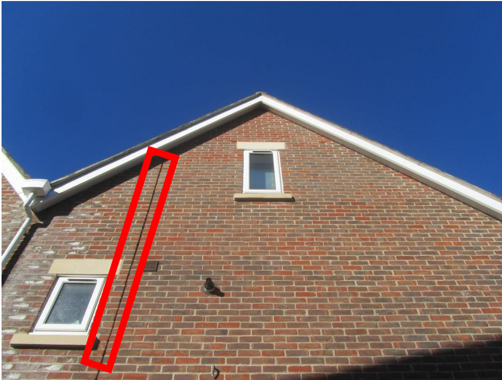
Photo 9 – View of expansion joint on the side elevation.
