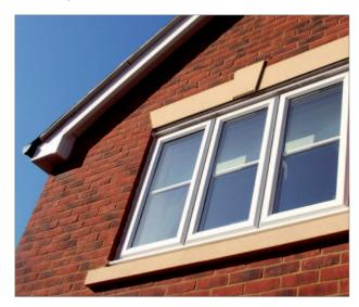
The material is recognised in NHBC Standards and the use of features made from cast stone should minimum comply with the latest version of BS 1217 or the higher standard adopted by members of the UKCSA.
